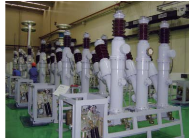
40.5kV SF 6 circuit breaker under commissioning
